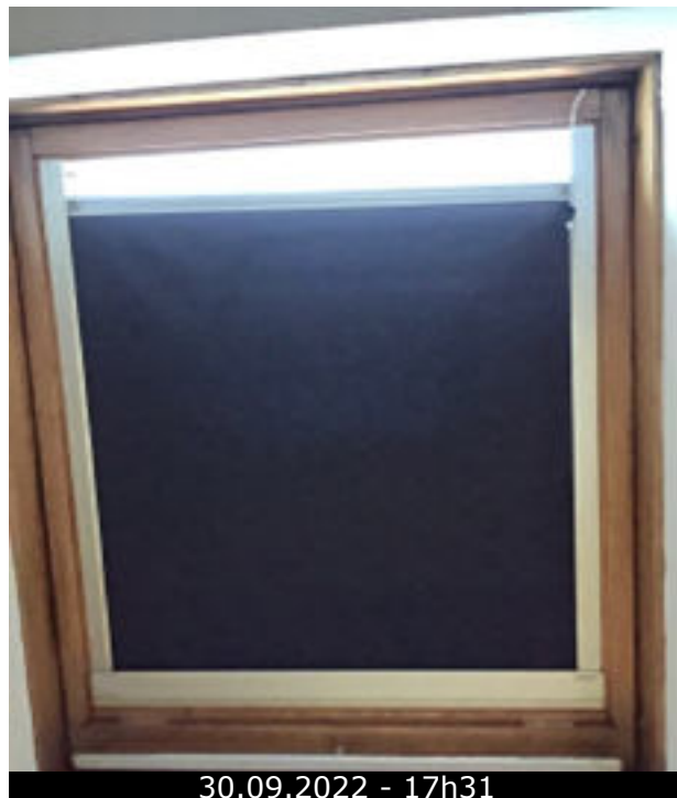
Photo 46 (Cuisine / Stores / Etat d'usage)
