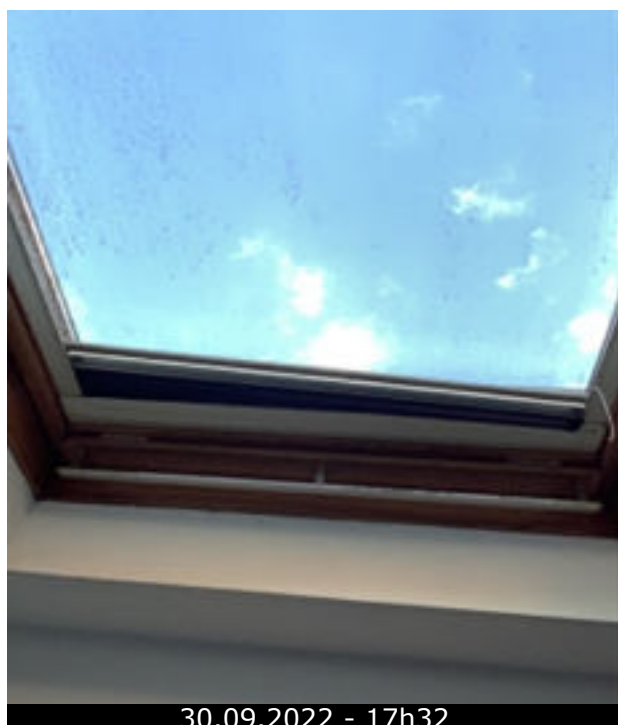
Photo 47 (Cuisine / Stores / Etat d'usage)
